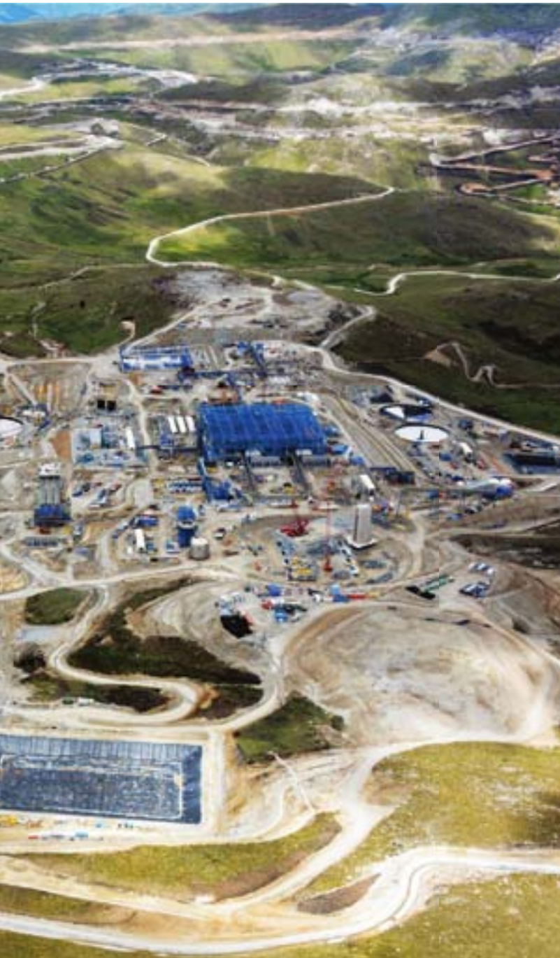
Tailings thickeners and concentrator, Las Bambas
